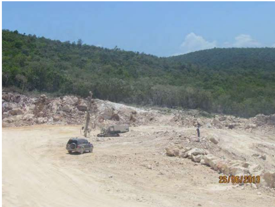
Plate 3: Drilling in the process of establishing benching
