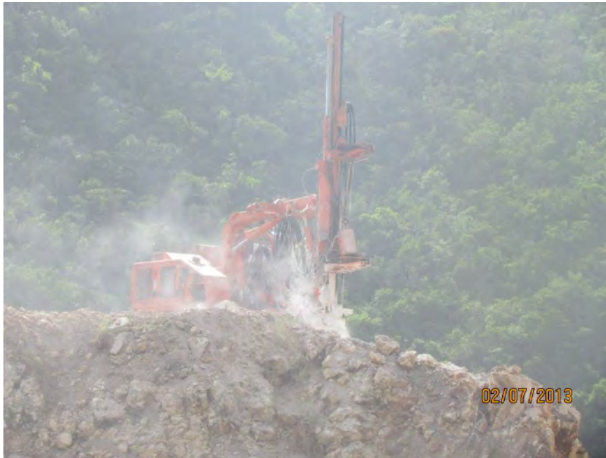
Plate 1: Drilling in Preparation for Blasting
