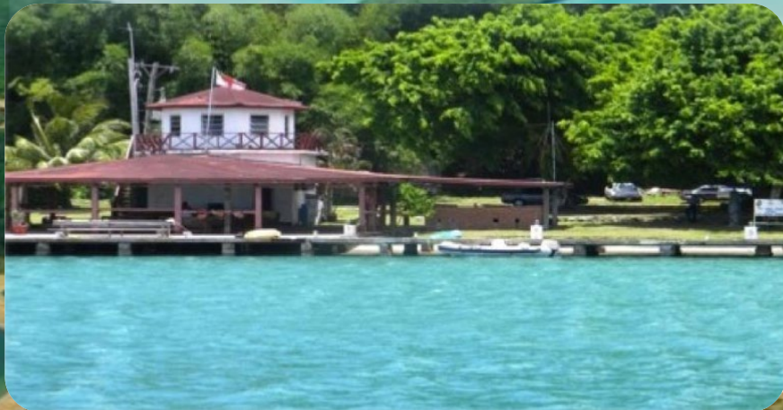
Bowden Coast Guard and Marine Police Facility
