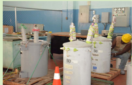
A worker at FTMCL apply the finishing touch to a transformer in the final stage of production.
